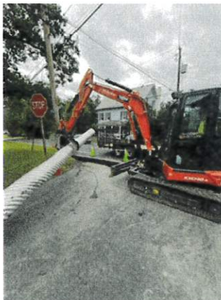
Pleasant View Road Pipe Replacement
