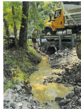
Pleasant View Road Once Cleaned Up
